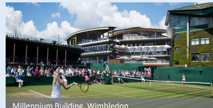
Millennium Building, Wimbledon
