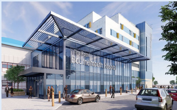
The Royal Bournemouth Hospital Status: On Site Current project Value: £17m Phase 2 opportunity: £8.5m
