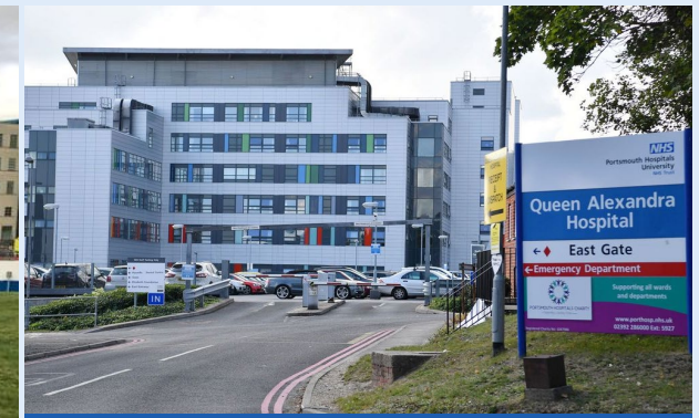
Queen Alexandra Hospital, Portsmouth HV Infrastructure upgrade Status: *PCSA £23k Project Value: £6m
